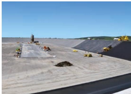
The power plant is being given a new sealing layer and its storage capacity increased by 70,000m<sup>3</sup> to prepare it for its future task of cancelling out fluctuations in power supplies
